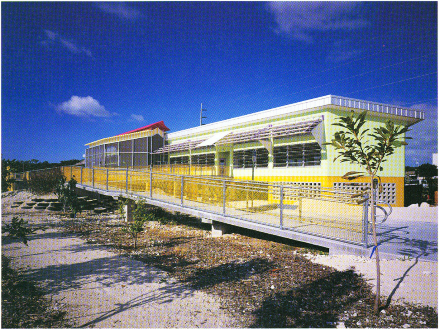
EXTERIOR VIEW—SOUTH SIDE
